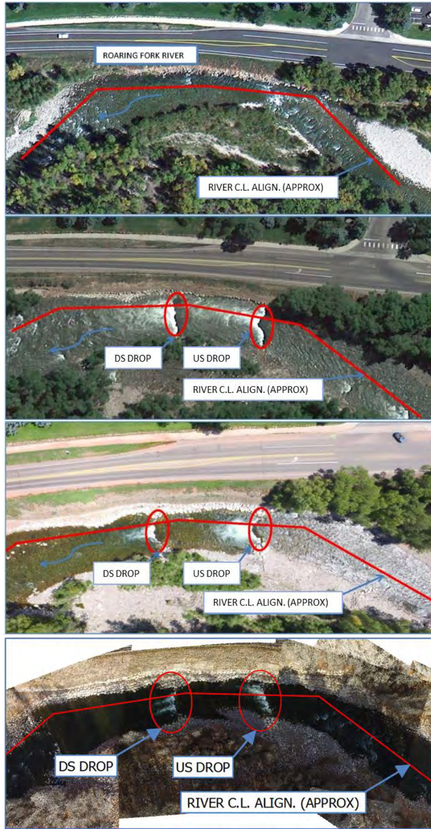
Figure 2. Pre-construction, post-construction, and post-runoff aerial photography of project site (September, 2011; June, 2017; August, 2017, November 2020, respectively) Upstream (US) and Downstream (DS) drops.
