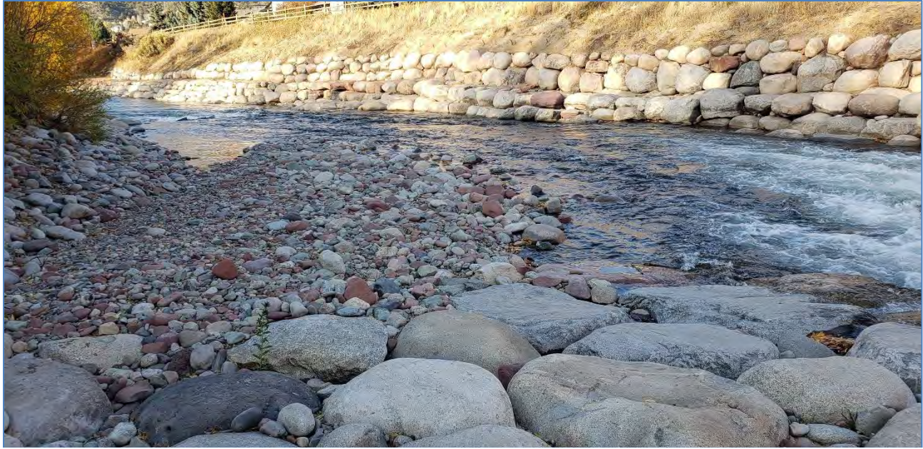
Figure 10. View from left wingwall of upper feature facing downstream. Newly formed depositional gravel/cobble bar.
